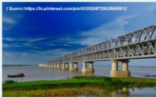
Digha-Sonpur Rail-Road Bridge
